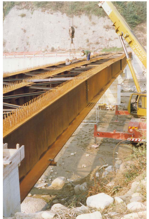
Figure 13: Composite bridge made of I-beams during assembly
